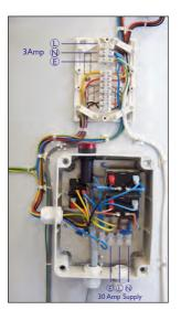
The higher immersion heater can be wired to a 15 amp switched spur for the householder to use as boost during periods of heavy hot water demand.
