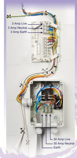
Full instructions are supplied with the unit for the plumbing and wiring. A dedicated 30 amp supply will be required for the 6kw immersion heater supply in addition to a 3 amp supply for the programmers and pump as shown above.
